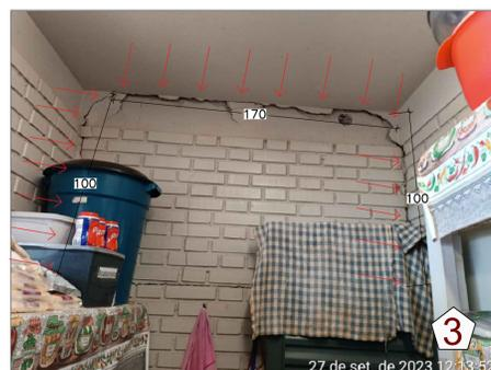
**IMAGEM DOS ELEMENTOS A SEREM TRATADOS COM ARGAMASSA EXPANSIVA SEM ESCALA**
