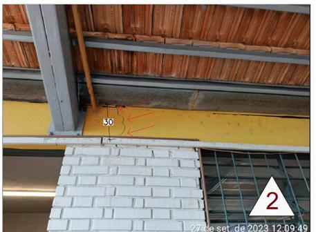
IMAGENS DAS VIGAS A SEREM TRATADAS COM RECOMPOSIÇÃO COM GROUT SEM ESCALA
